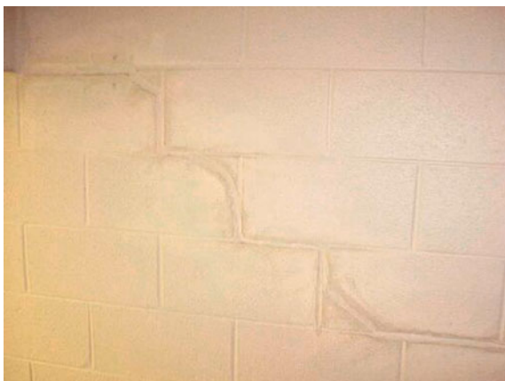
Fig. 13 Repaired masonry block cracks
