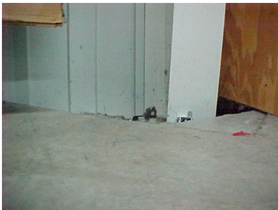
Fig. 24 Heaved floor adjacent to load-bearing wall on main floor of the Carhartt Factory. Note the cell phone resting on steel column for scale
