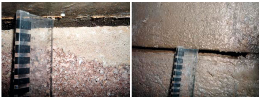
Fig. 73 Rise of a manhole biscuit/cover slab of up to 13 mm due to the expansion of the surrounding pyritiferous fill ( left ). In the manhole wall itself gaps of up to 10 mm were noted ( right ) where the upper wall remained cemented to the biscuit
