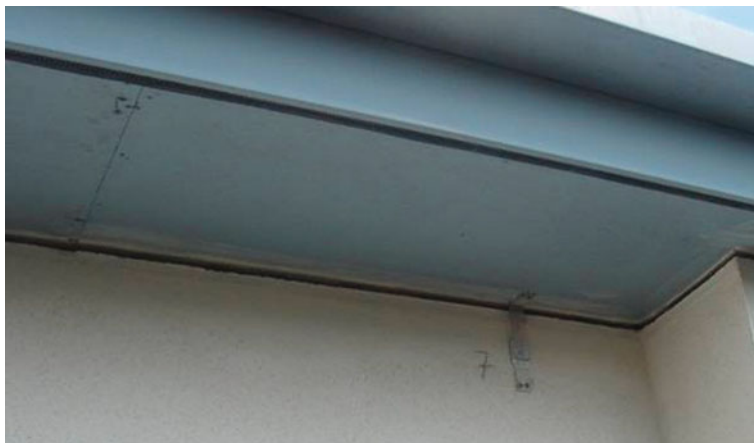
Fig. 20 Gap of some 40 mm which developed at eaves level within 5 years of construction
