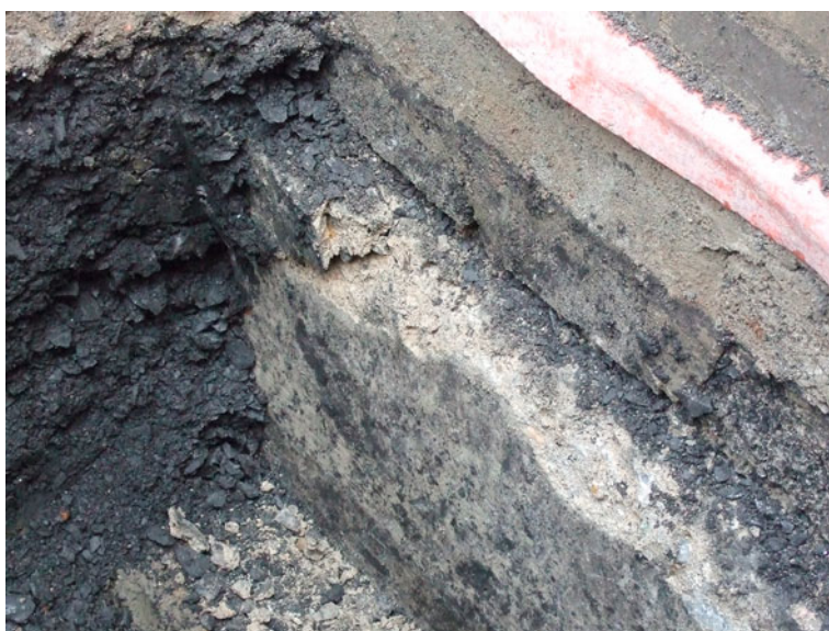
Fig. 28 Deterioration of concrete at the top of the beam, TP 11, and the nature of the dark deleterious fill adjacent to it
