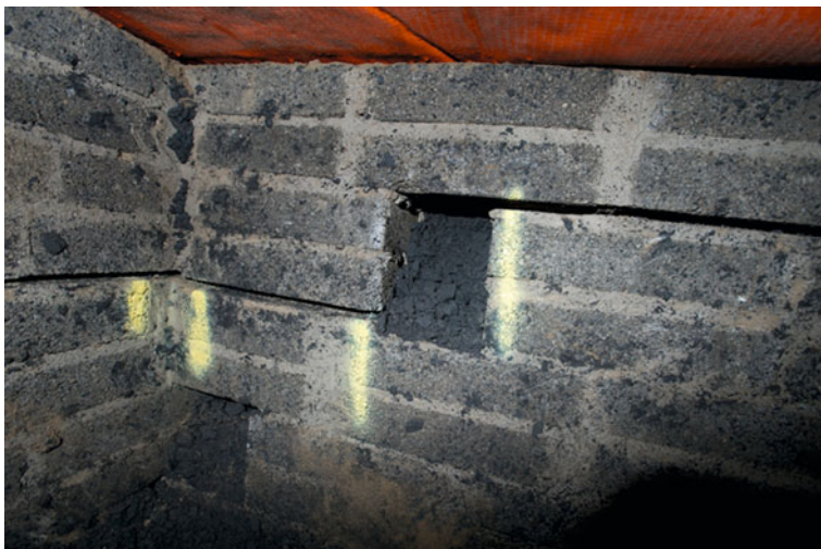
Fig. 7 Horizontal gaps (up to 20 mm) observed in a rising wall immediately after the fill was removed in a localised trial pit (the balance of the fill beneath the floor slab was still in place at this time)
