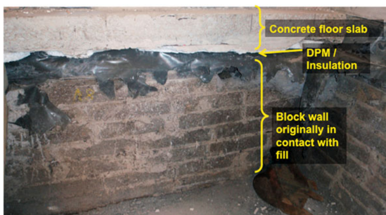
Fig. 18 Exposed internal foundations constructed from concrete blocks on a concrete footing
