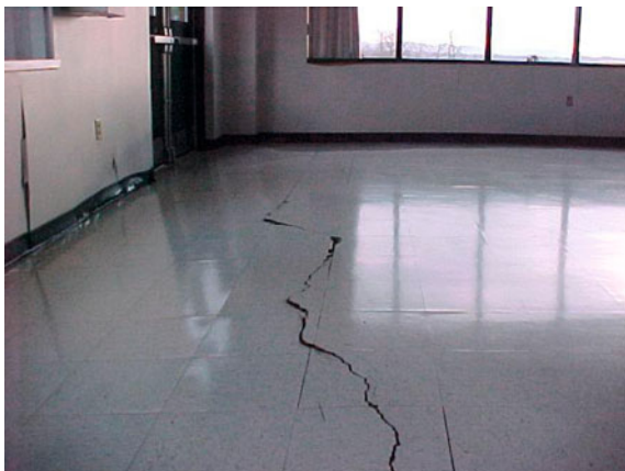
Fig. 22 Substantial floor cracks in Carhartt break room; rise of walls has caused the window to be inoperable
