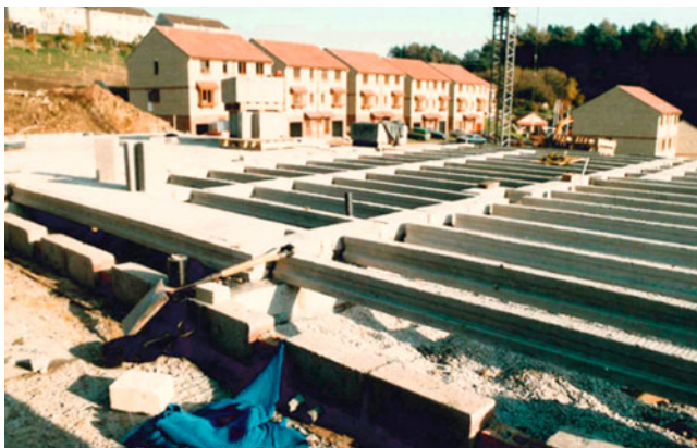
Fig. 45 Suspended floor slabs recommended for houses constructed over pyrite-rich Westbury Beds at Radstock, N Somerset
