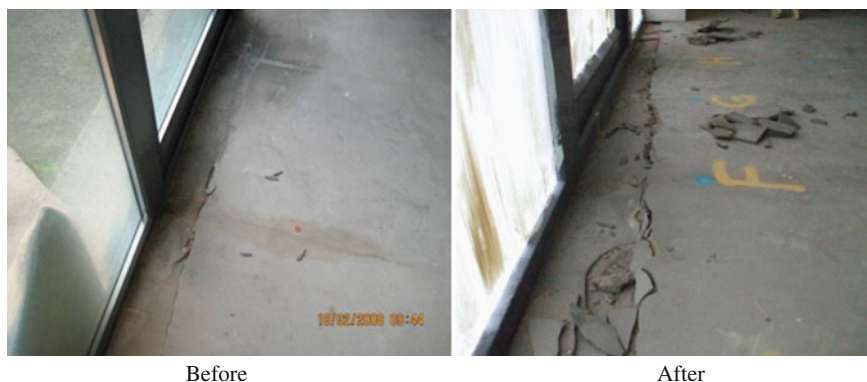
Fig. 6 Effect on the ground-bearing floor slab after the removal of fill in an adjacent property
