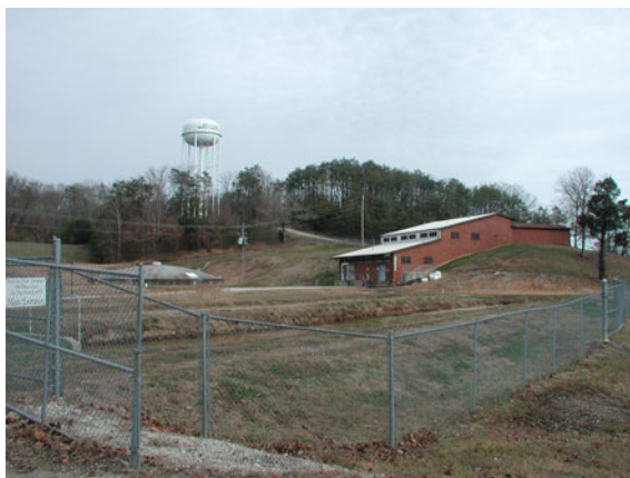
Fig. 29 Clay City (Beech Fork) Water Treatment Plant
