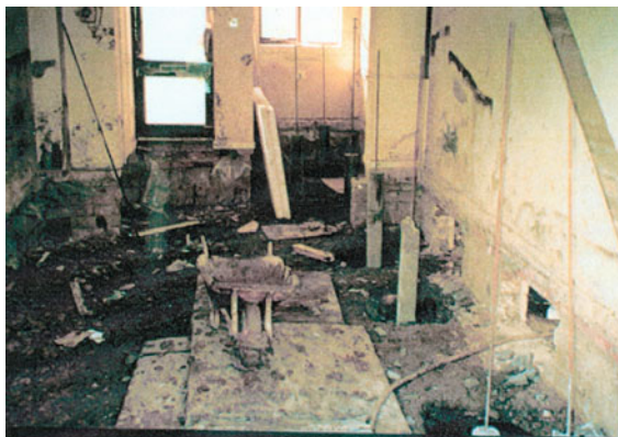
Fig. 49 Remediation included installation of piles to support suspended floor slabs at Hucclecote
