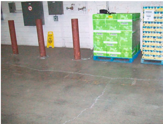
Fig. 12 Intersecting floor cracks indicative of upward heave of the slab
